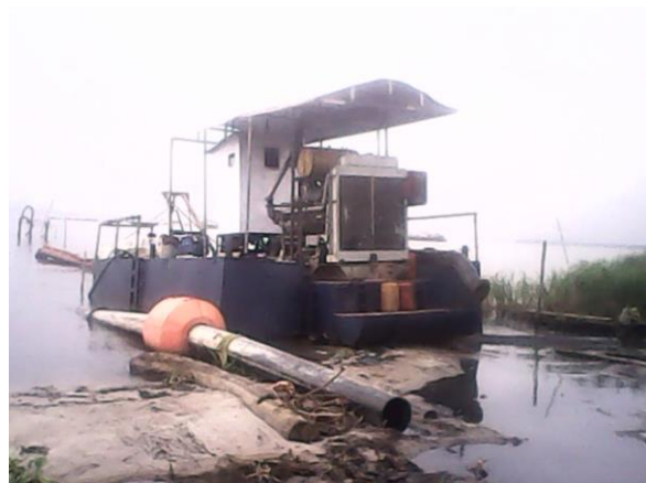
Intensive dredging activity in Epe
