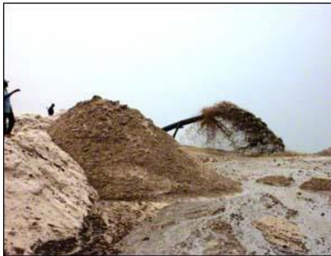
Ongoing dredging activity
